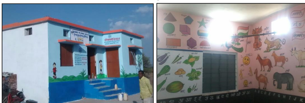
Renovated AWC in Lamba Talab village
